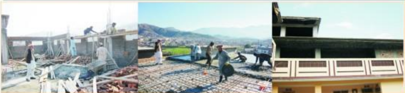
Residential Rooms under construction at KKF Girls Campus
